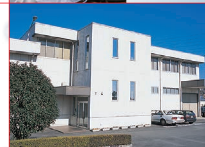
The Takasaki Plant (Custom Manufacturing Operations for Cosmetics)
